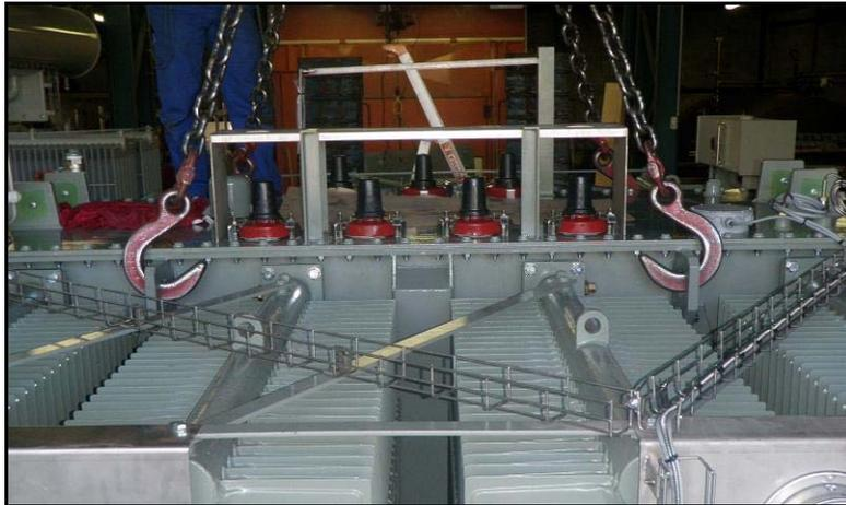
When unloading, the rollers must be mounted on the substructures and tilted in the desired direction. The yokes are stopped from turning using the envisaged screws.
